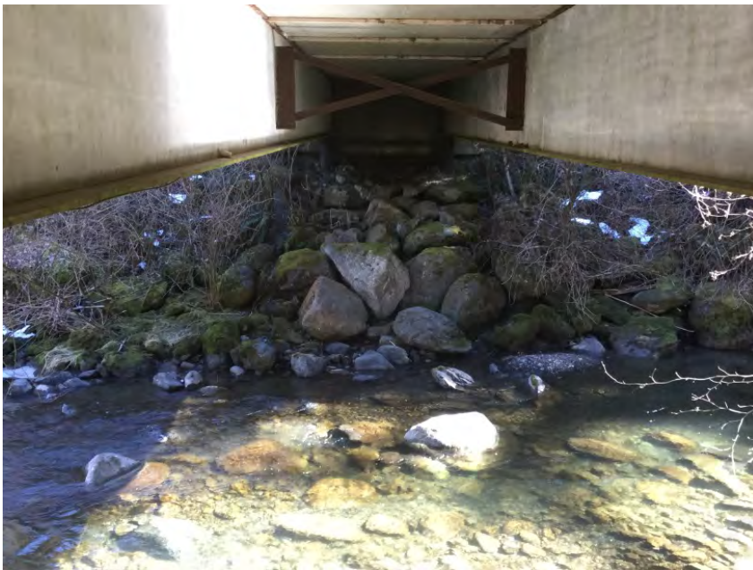
Right Bank Abutment when facing downstream
