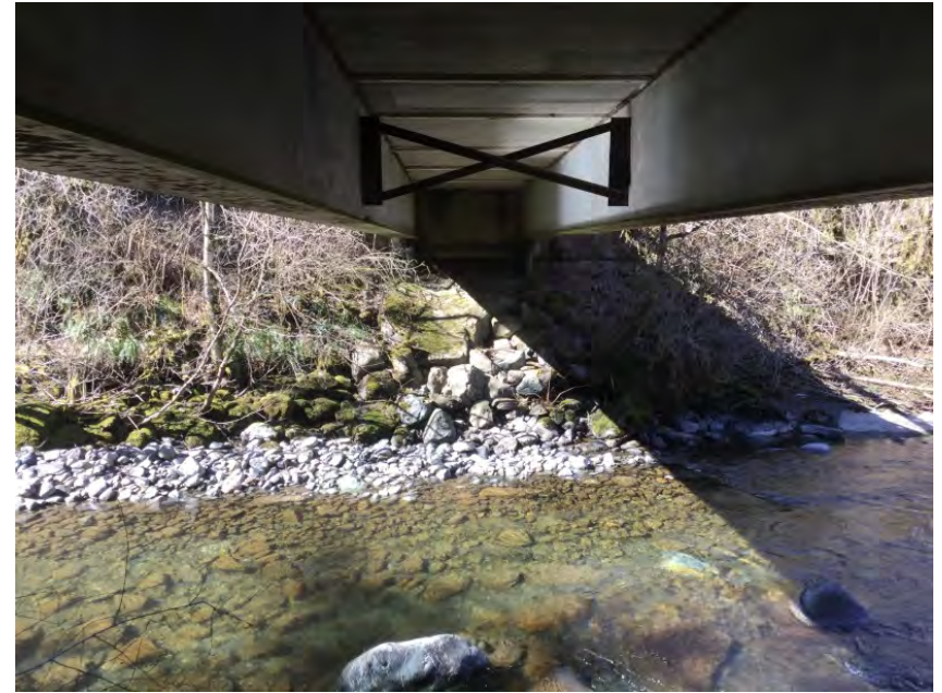
Left Bank Abutment when facing downstream
