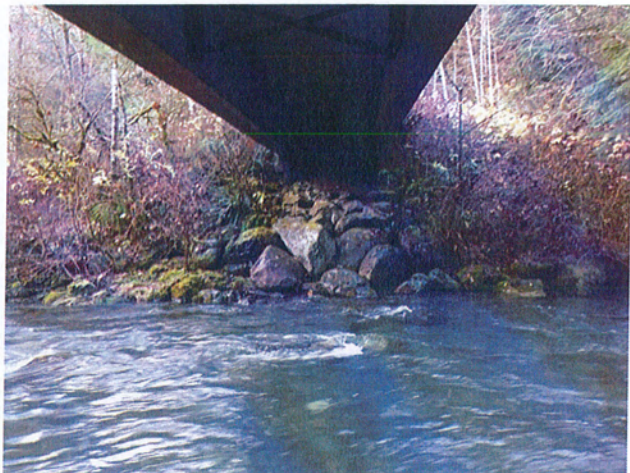
Right Bank Abutment when facing downstream
