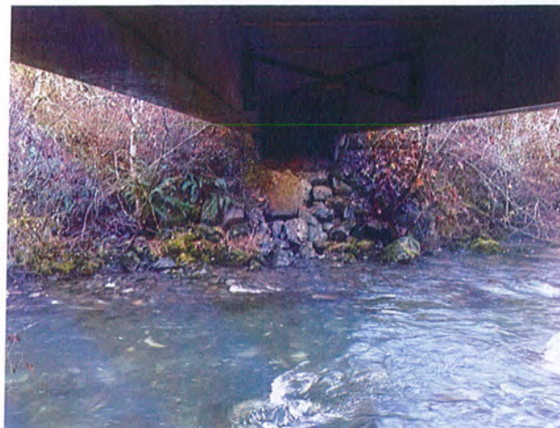
Left Bank Abutment when facing downstream
